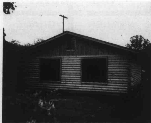
Main Street View of New Annex
